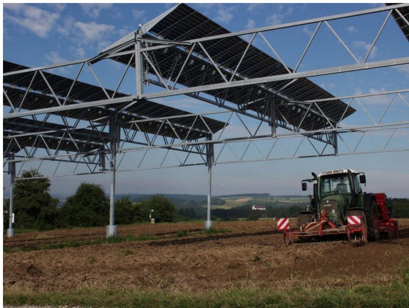
Figure 2: Agro-photovoltaic system of the Hofgemeinschaft Heggelbach 14 . Agricultural production and energy production in the same place are not mutually exclusive.
